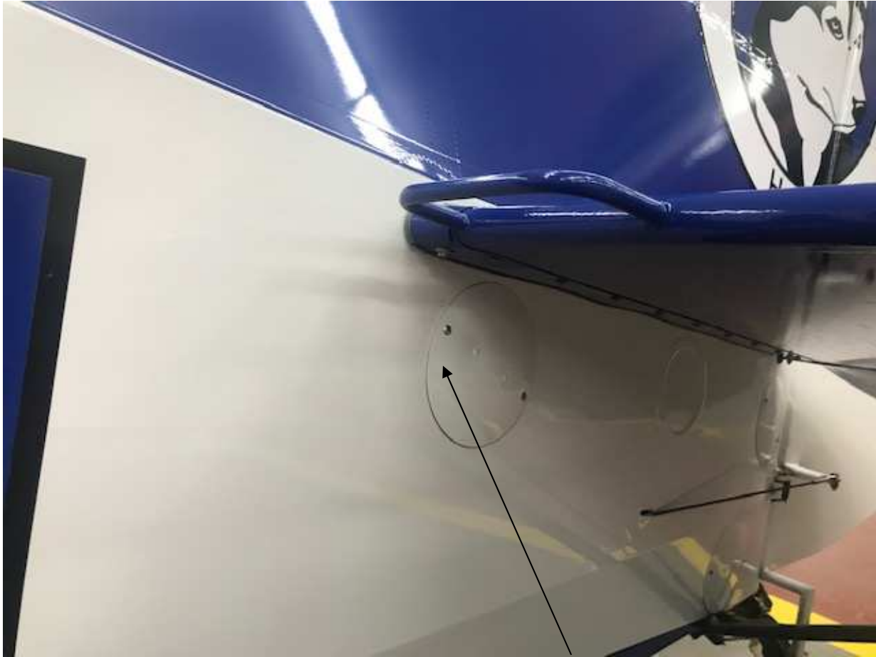
Figure 2, Inspection access hole cover LH side
