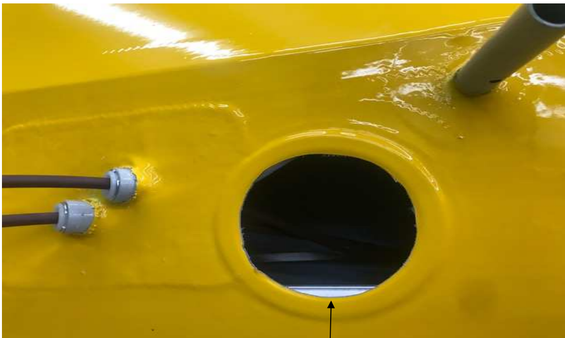
Figure 4, Cut out inspection ring
